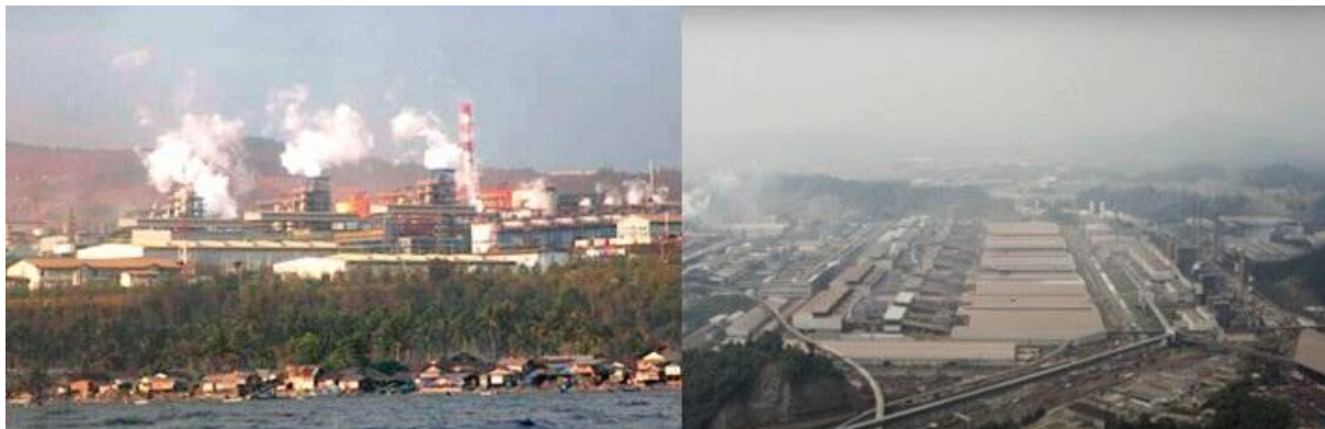
Figure 4. Nickel industrial area
